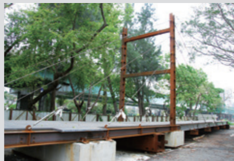
▲ A lightweight transportable emergency bridge made of composite materials
