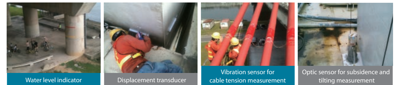
▲ On-site installation of monitoring system instruments
