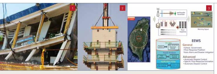
In-situ experiment of existing school building 2 The precast segmental post-tensioned concrete bridge column 3 Diagram of Earthquake Early Warning System (EEWS)
